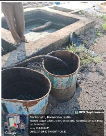
Oil collected in drums from At the inlet of ETP
